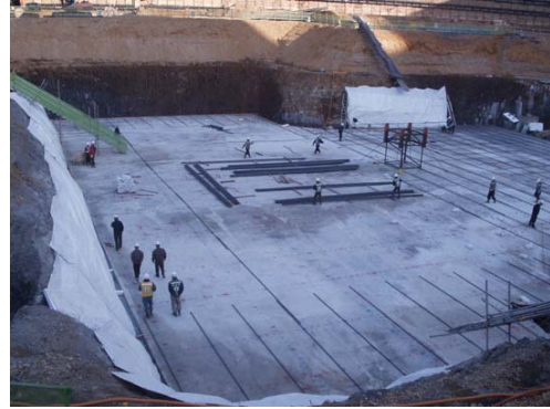
Fig. 8. Preparation of Mat Construction
