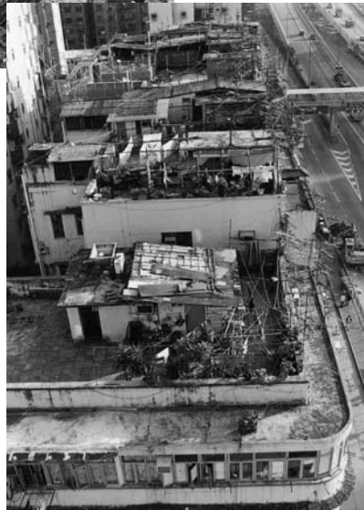
Figure 5 Illegal structure constructed on the roof top of some post-war buildings in Yaumati District of Kowloon.
