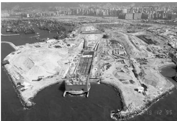
Figure 16 Coupling arrangement and approach ramp for the Western Harbour Crossing on the south-most tip of the West Kowloon Reclamation.
