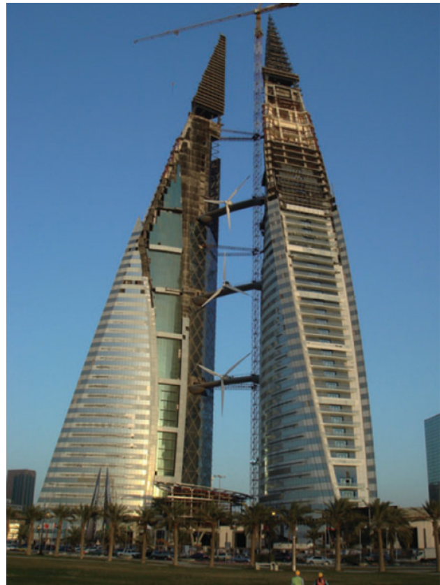
Figure 10. Bahrain World Trade Center, Manama. In recent years the exploitation of on-site energy generation from renewable sources has become a common characteristic of fifth generation tall buildings. [Source: Smith & Killa, 2007]
