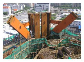
Figure 6. The diagonals of the mega-structure, formed from welded boxes of structural steel.
