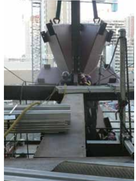
Figure 15. Placing of the atrium node. © Yolles
