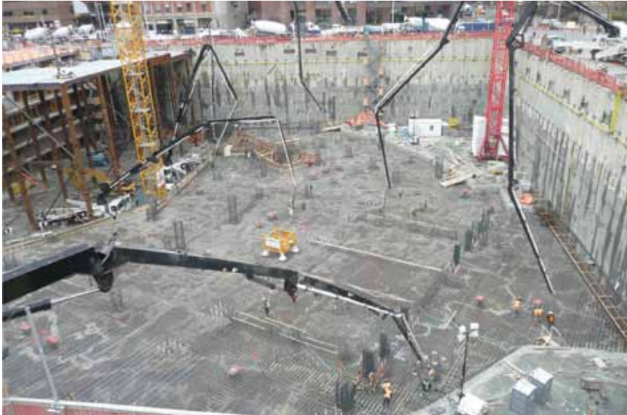
Figure 14. Commencement of the raft pour. © Yolles
