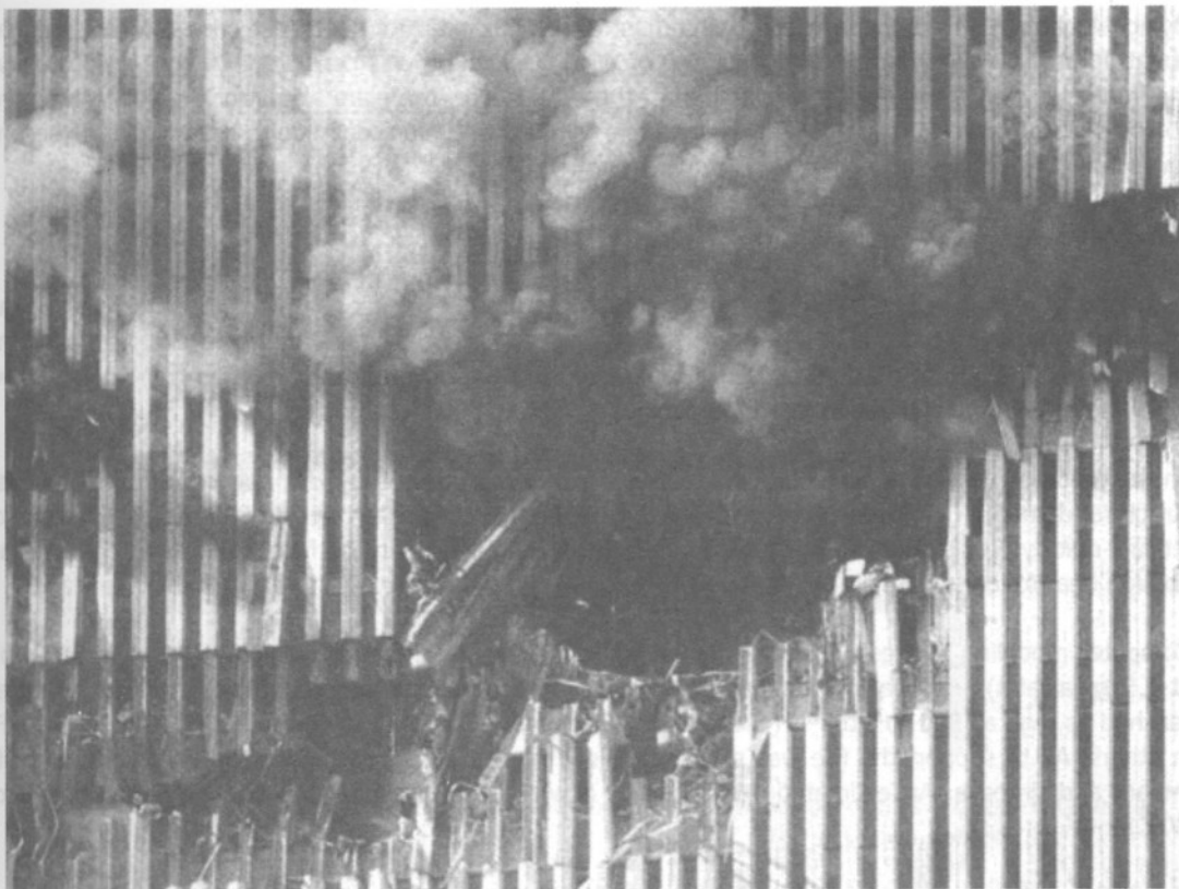
Fig. 2. Impact damage to the north face of WTC1
