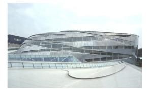
**Fig. 4.** Ribbon shaped glass zones cross the roof of the new town hall of Alphen aan de Rijn (NL)
