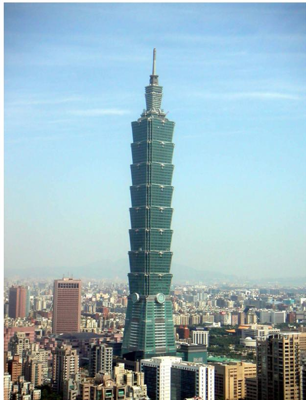
**Fig. 1.** The Taipei 101 profile shows a truncated pyramidal base topped by eight, 8-story flaring building modules, a narrower equipment/observation deck module and a steel-spined spire
