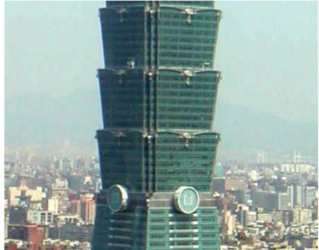
**Fig. 3.** A close-up of the tower corner clearly shows the ‘sawtooth’ treatment above Floor 25 for wind vortex reduction.
