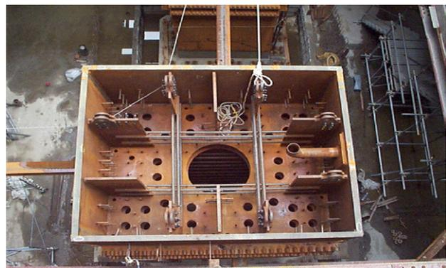
Fig. 6. A supercolumn box just below its field splice location. High strength concrete enters through the pipe at right to fill the box from bottom up in two-story lifts.
