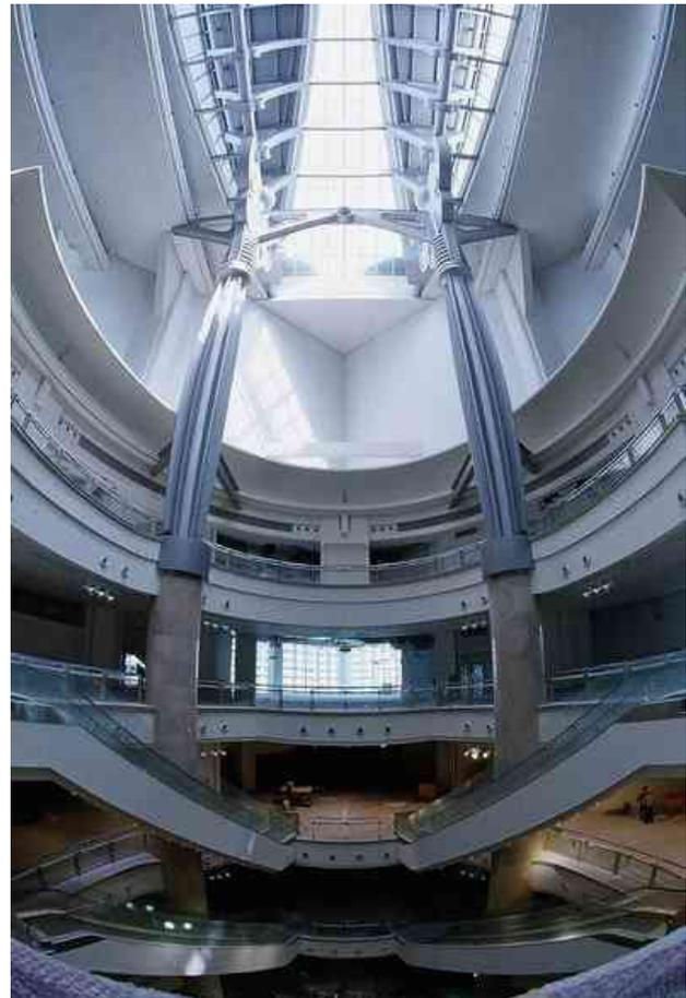
**Fig. 12.** Twin Vierendeel trusses span the shopping mall atrium within the building podium.
