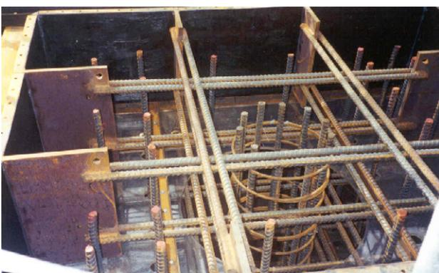
**Fig. 8.** Concrete fill is reinforced by vertical bars threaded through diaphragm holes and a spiral-wrapped core threaded through the central manhole.
