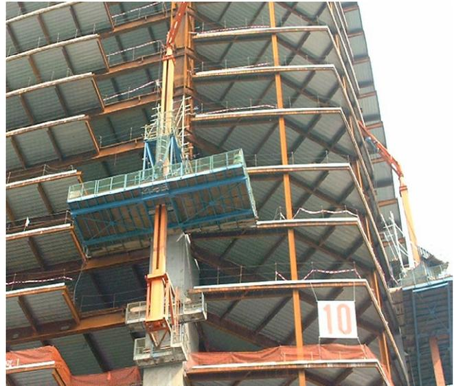
Fig.4. Column Climbform System
