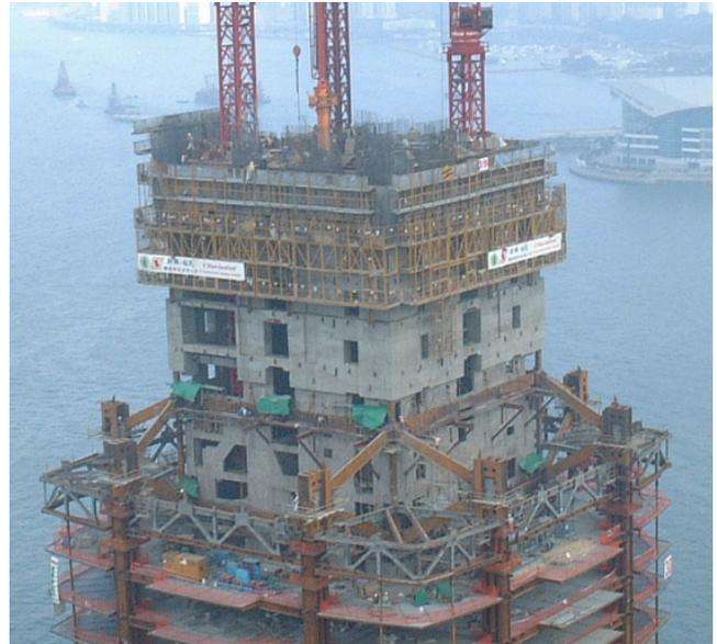
**Fig. 8** Climbform construction of the core progressing prior to completion of the steel outriggers.
