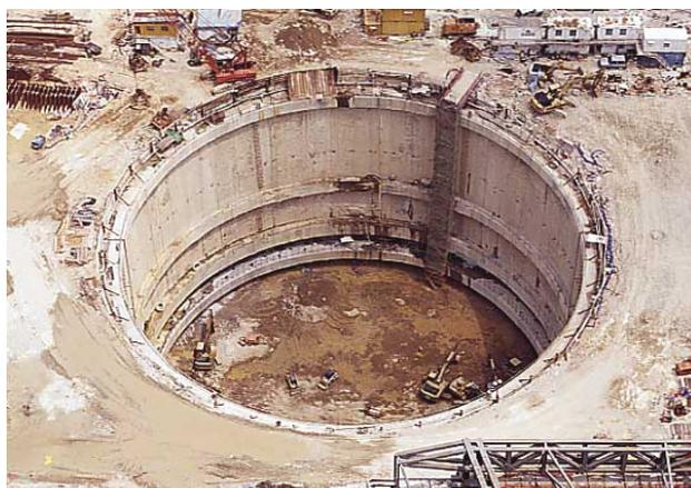
**Fig.2.** Excavation within the temporary cofferdam
