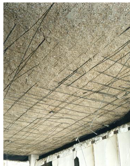
Figure 11 Spalling of concrete floor slab following the Cardington fire test.
