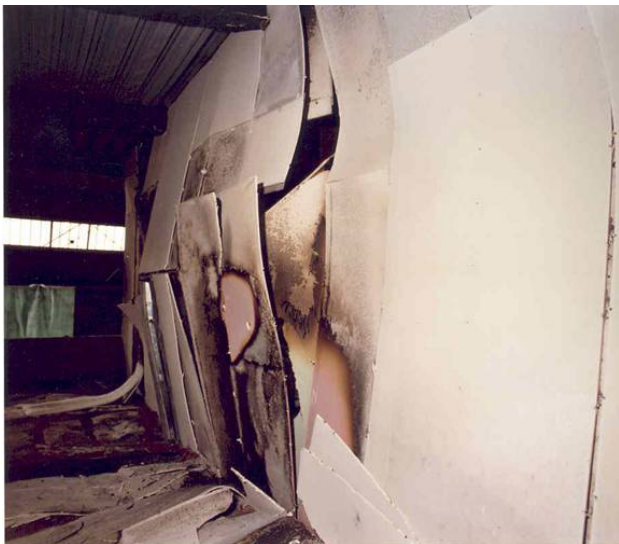
Figure 2 Failure of non-loadbearing compartment wall due to deformation of the structure.
