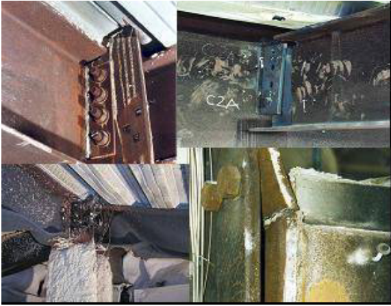
Figure 9 Fracture of end-plates and shear failure of bolts in various connection types following a fire.
