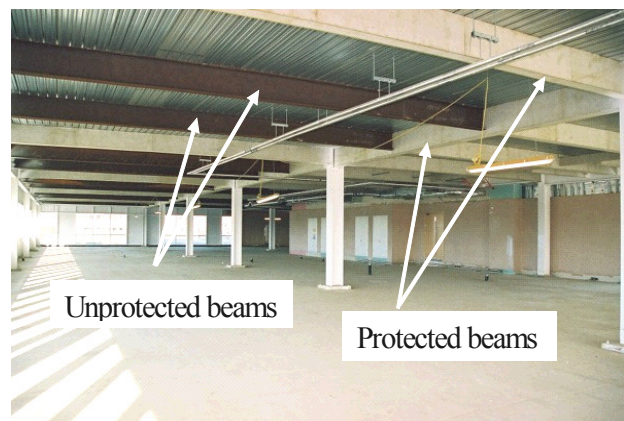
Figure 8 Example of using membrane action in the floor slab.
