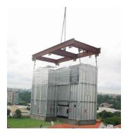
Figure 4: HDB's Prefabricated Boxed-Toilet
