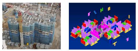
Figure 2: Fully Precast System used for super high-rise construction
