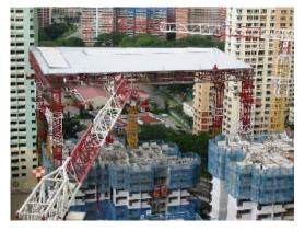
Figure 6: Automatic Building Construction System (ABCS)
