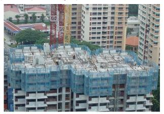
Figure 5: Climbing Safety Working Platform used to enhance safety on site.
