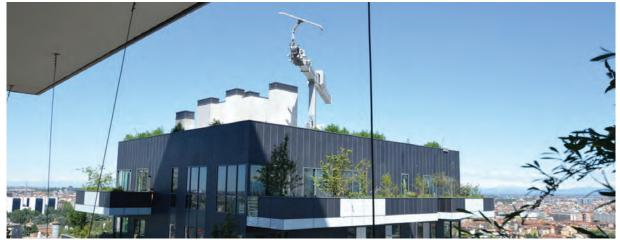
Figure 7. Telescopic arm on the roof of Tower D The arm should drop the maintainers from the outside of each tower. 图7. D座屋顶伸缩臂 维护电梯由伸缩臂从每个塔外部降下。
