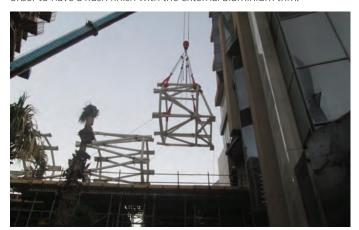
Figure 5. Erection of bridge module (source: AGC-A) 图5. 桥模块的安装 (出自AGC-A)
