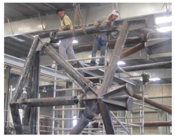
Figure 4. structure pre-assembly in the steel workshop (source AGC-A) 图4. 车间内的预组装结构 (出自AGC-A)
