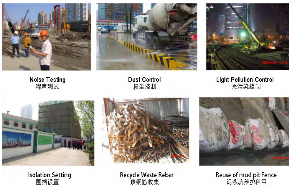
Figure 2.19. The environmental control during the construction process of Shanghai Tower (Source: Shanghai Research Institute of Building Sciences.)
