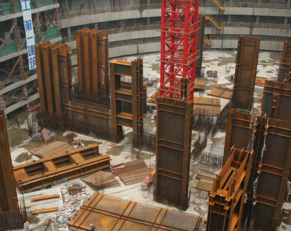
Figure 5.15. The heavy steel structure of the Shanghai Tower in its early stages (Source: Antony Wood) 图5.15. 上海中心施工初期的重型钢结构 (来源: 安东尼·伍德)
