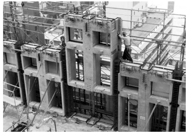
Figure 20. A view of installation of exterior PC panels.
