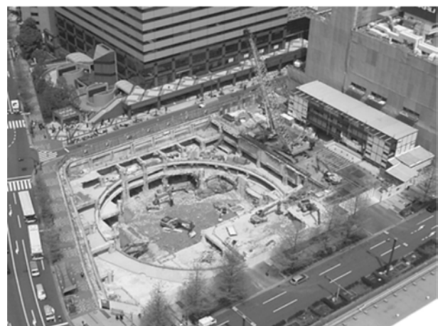
Figure 12. Construction simulation for underground works using RC ring beam.
