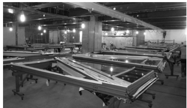
Figure 15. Pre-assembling of curtain-wall units at site factory.
