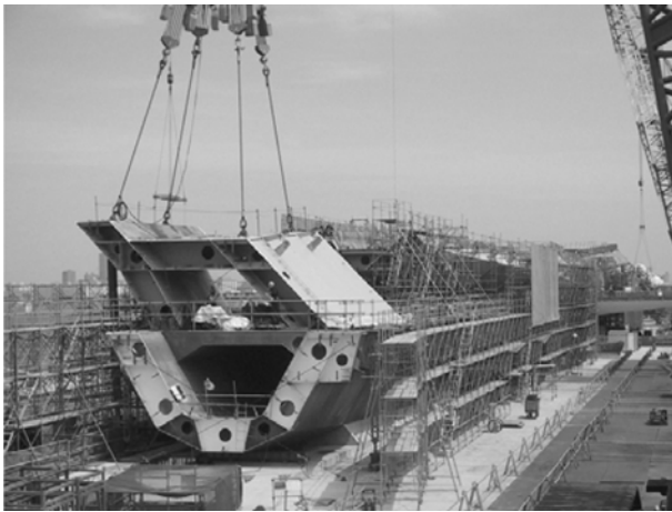
Figure 6. Construction by large steel blocks.
