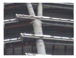
Photo 2. Cast steel connection for peripheral tilted column-crossed section.
