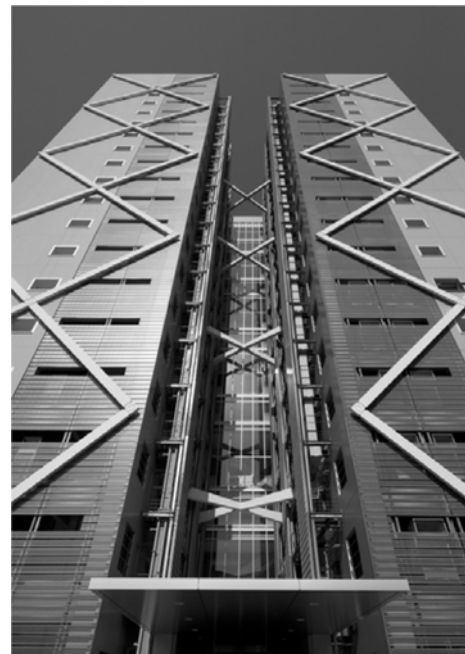
Figure 20. Mega-Brace elevation from south side.
