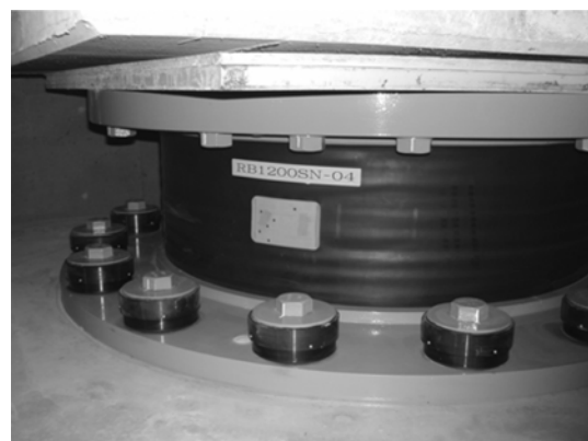
Figure 12. Setting of spring washer.
