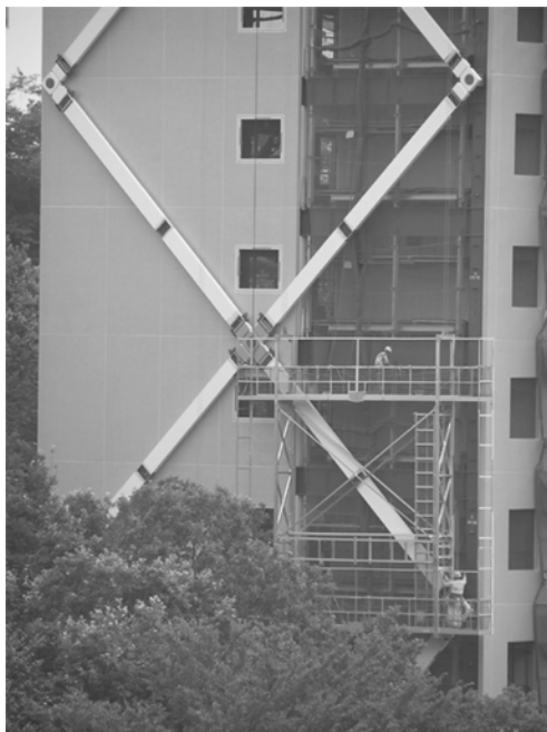
Figure 18. Construction of Mega-Brace.
