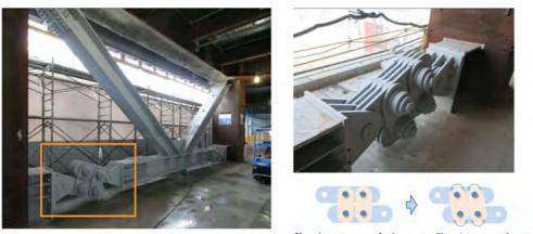
Figure 28. Appearance of rotational friction damper.
