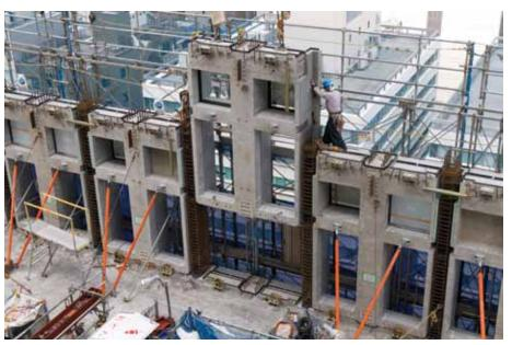
Figure 12. Installation of perimeter precast frames.
