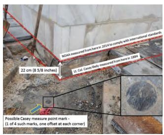
Figure 4. Illustration of the measuring points used by Lt. Col. Thomas Casey in 1884 and the 2014 measuring point used by NOAA to meet CTBUH standards.
