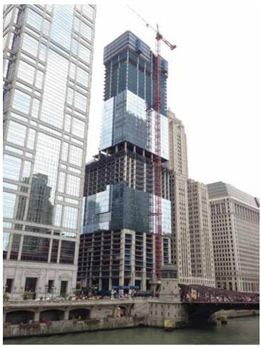
Figure 13. Curtain wall installation in two, later three stacks with three separate crews (Source: Handel Architects)
