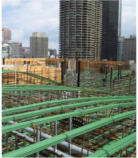
Figure 8. Transfer matt before first pour (Source: Handel Architects)
