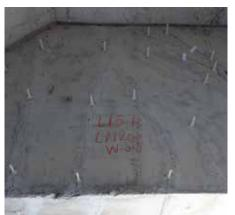
Figure 2. Diagonal shear cracks and vertical flexural cracks in perimeter girders under slanting column and dummy column location at Level 16 (Source: Daewoo E&C)
