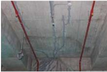
Figure 4. Cracks on the soffit of floor slab at Level 16: cracks in non-rectangular slab (above) and slab cracks connected with cracks in a perimeter girder (below) (Source: Daewoo E&C)
