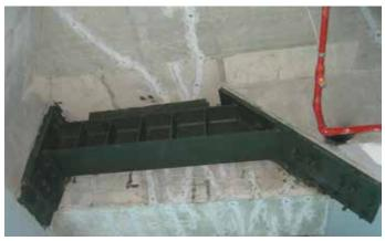
Figure 15. Cracked perimeter girder reinforced with steel member (Source: Daewoo E&C)
