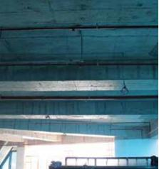
Figure 6. Cracks on the side of perimeter girders (above) and beams connecting perimeter girders and core walls (below) at Level 16 (below) (Source: Daewoo E&C)
