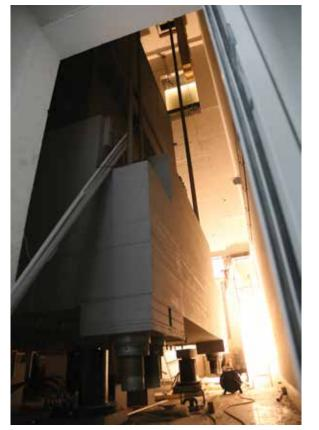
Figure 19. Tuned Mass Damper of the DCT 1 (Source: Bollinger + Grohmann)
