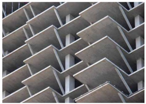
Figure 5. Slabs at the Folded Façade (Source: Bollinger + Grohmann)
