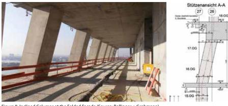
Figure 8. Inclined Columns at the Folded Façade (Source: Bollinger + Grohmann)
