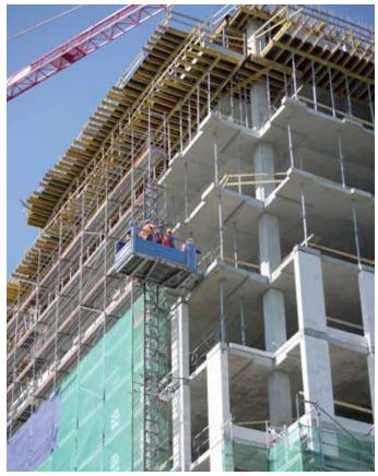
Figure 5. An external hoist exposes construction workers to the elements and must be shut down in severe weather due to safety concerns (Source: Shutterstock/pryzmat)
