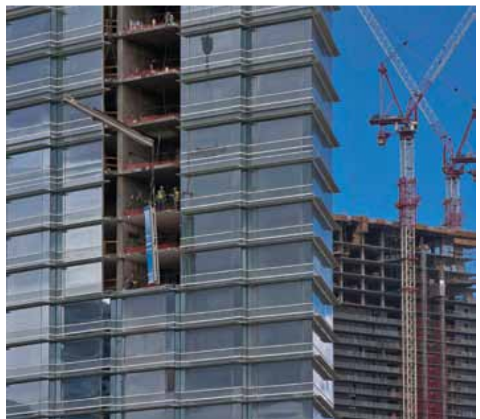
Figure 3. The prefabricated modules of a unitized façade system speed the erection process. (Enclos Corp)
