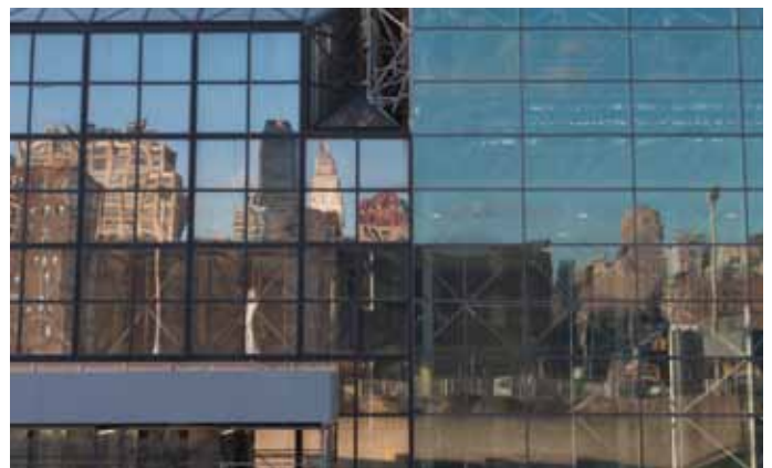
Figure 4. IGUs in place since the mid 1980s are currently being replaced at the Javits Convention Center in New York City (new units to the right). (Enclos Corp)
