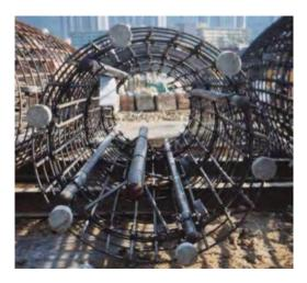
Figure 3. Reservation pipe within bored piles.
