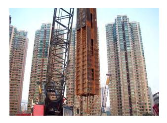
Figure 13. Stanchion installation into Bored Pile.
