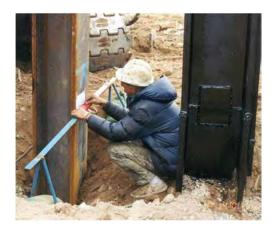
Figure 7. Final setting of pile.
