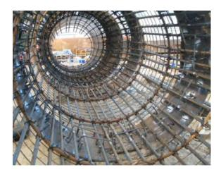
Figure 12. Steel Collar in the Bored Pile.
