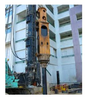
Figure 6. Pile pitching using hydraulic hammer.
