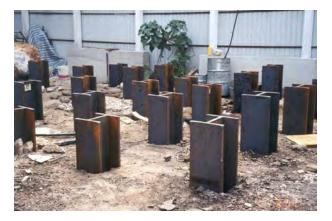
**Figure 5.** Snapshot of a site using percussive steel H-pile foundation.
