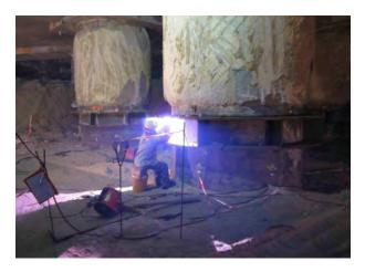
Figure 21. Welding of bracket for beam/slab reinforcement connection.
