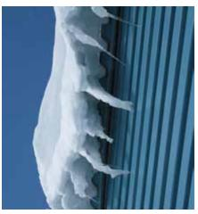
Figure 3. Example of hazardous ice formation on a ledge. © NMI
