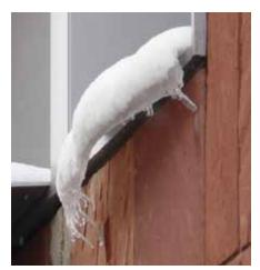
Figure 2. Example of hazardous ice formation on window sill. © NMI
