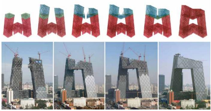
Figure 9: CCTV construction sequence. © Arup
