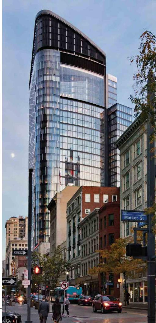
ventilation and thermal stack effect ventilation strategies were considered; the latter was chosen as a more controllable option, both at the scale of the entire building and on the individual floors. The strategy intended to introduce negative air pressure at the façade, so fresh air would be drawn into the building, and up through a central shaft. This was validated with extensive computational fluid dynamics (CFD) modeling at the early stages of design.
