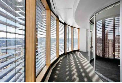
Figure 14. Wooden mullions provide embodied energy savings and a unique, enhanced aesthetic. @ Connie Zhou Photography
