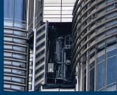
Instead, a unique combination of mobile, wall-mounted machines was designed specifically for this application. The solution consists of three wall-mounted machines located at each of levels 40, 73 and 109 (nine in total). These complex machines launch from within their internal parking space through a retracting panel, and travel along a set of tubular stainless steel rails.
