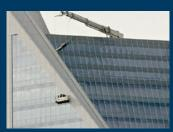
In order to reach all parts of the building including the extreme corners, the five-stage jib assembly is capable of luffing up to a maximum angle of 60 degrees when at maximum outreach.
