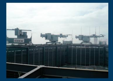
One of the three systems was designed with an articulated cherry-picker extension to provide personnel access to the helipad on the roof of the skyscraper, as well as conventional façade access.
