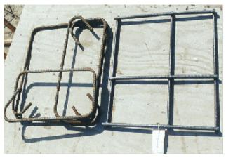
Figure 2 – Photo showing conventional reinforcement on left, WRG on right. (Baumann Research and Development, 2000)
