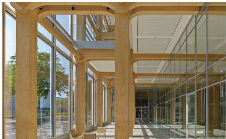
Figure 6. The Tamedia Office Building by Shigeru Ban Architects in Zurich, Switzerland, features a timber main structural system rising seven floors. Composite timber beam structures can achieve heights of 50-meters or more. (Source: Shigeru Ban Architects)
