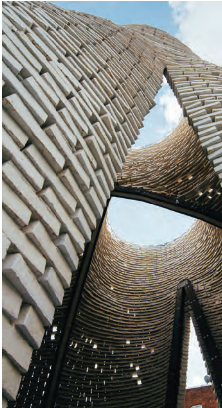
Figure 2. Hy-Fi, an installation by New York architects The Living, is the first tall structure built with bricks "grown" from mushrooms. (Source: David Benjamin) 图2. Hy-Fi是第一座用真菌砖垒成的高塔，由纽约The Living建筑事务所设计。（来源：David Benjamin）
