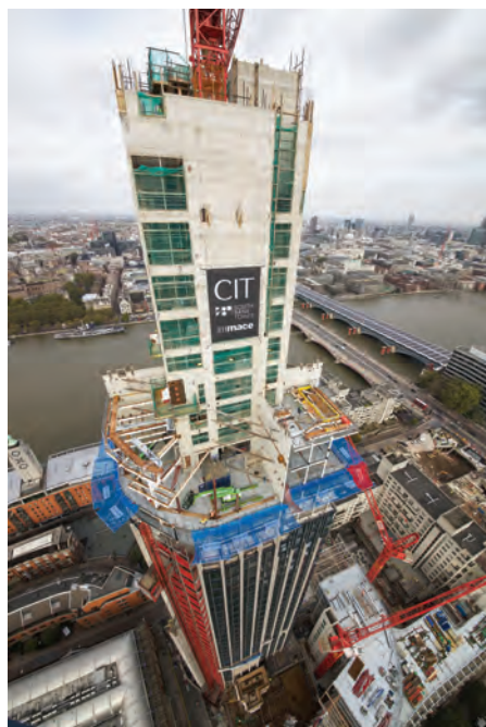
Figure 6. Site photograph of completed core (Source: Central Photography)
