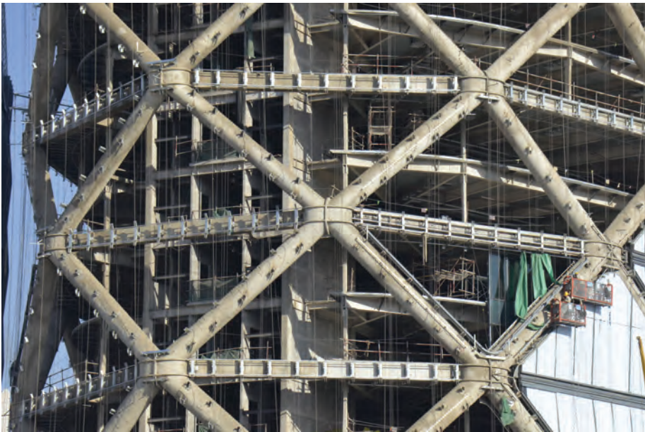
Figure 1. The Poly Diamond Lantern Tower is diagrid structure in Beijing, China. It uses a concrete filled steel tube frame which is a type that is particular to Asia. (Source: Terri Meyer Boake)
