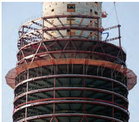
Figure 4. The composite system comprised of a reinforced concrete core with steel framing for the columns and beams can be adapted to different forms. It is not confined to orthogonal construction. (Source: Terri Meyer Boake)
