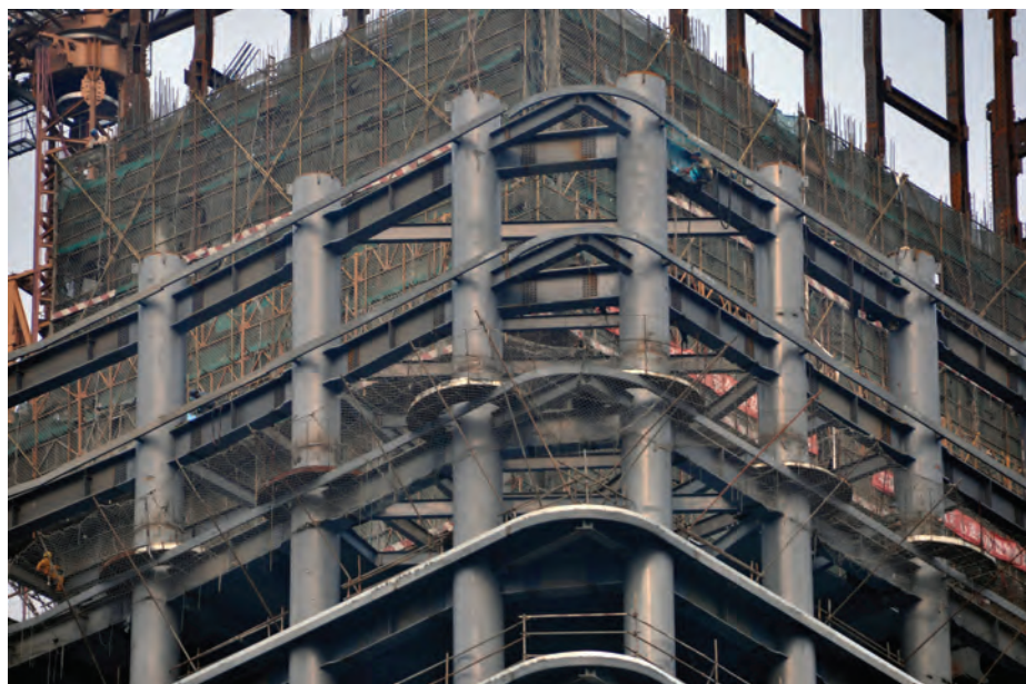
Figure 11. Concrete filled steel tube systems as constructed in China require a very high amount of site welding that would be unusual in Western markets. (Source: Terri Meyer Boake)
