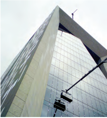
Figure 4. Example: extending cradle accessing deep recess (Source: Cox Gomyi) 图4. 拓展吊篮触及深凹处示例 (来源: Cox Gomyi)
