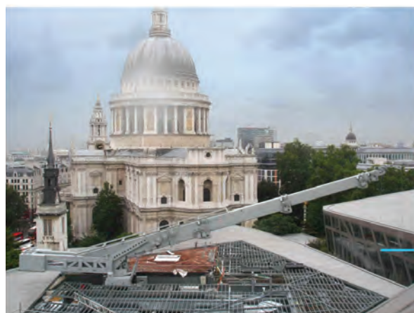
Figure 8. Example: BMU capable of parking below roof (Source: Cox Gomyi) 图8. 可停放于屋顶下的BMU (来源: Cox Gomyi)
