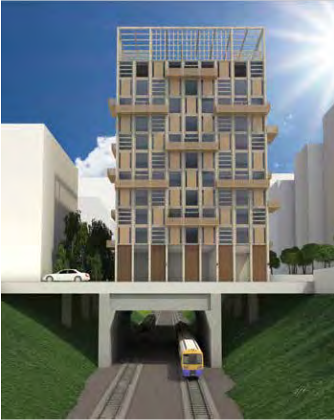
Figure 3. Schematic illustration of a 12-story flexible overbuild above rail tracks. © WSP
