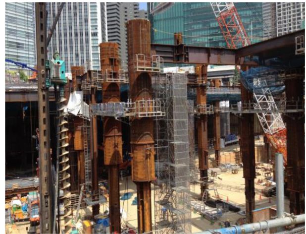
Figure 12. Construction of CFT Long Columns.
