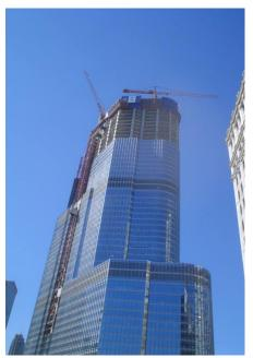
Figure 8. Trump Tower south elevation crane and construction elevator access
