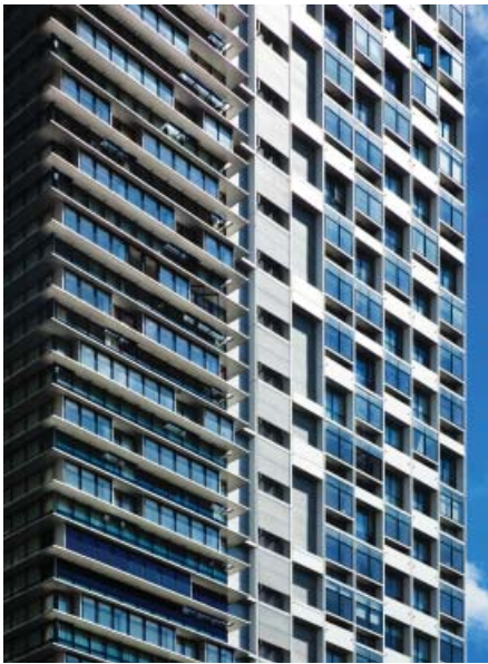
Figure 4. Moulmein Rise: The façade incorporates monsoon windows in the bay window ledges. Façade variations produce an interesting effect. © Patrick Bingham-Hall
