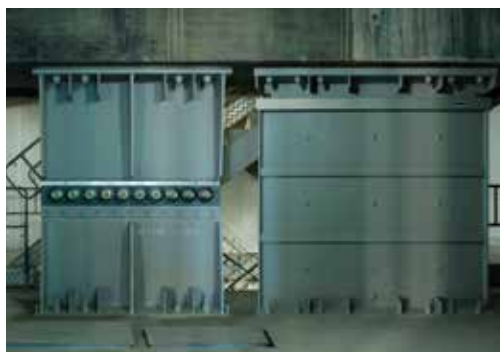
Figure 16. Viscous damping walls use steel plates attached to an upper and lower beam, with a viscoelastic material between them, at Ark Hills Sengokuyama Mori Tower, Tokyo. © Obayashi Corporation
