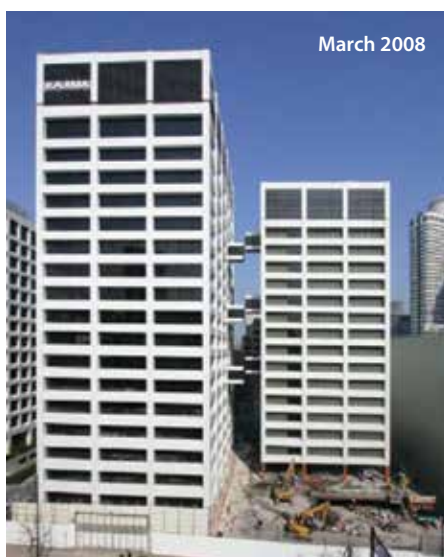
Figure 11. Kajima Cut & Take Down (C&TD) method, used on Kajima's former headquarters in Tokyo. © Kajima
