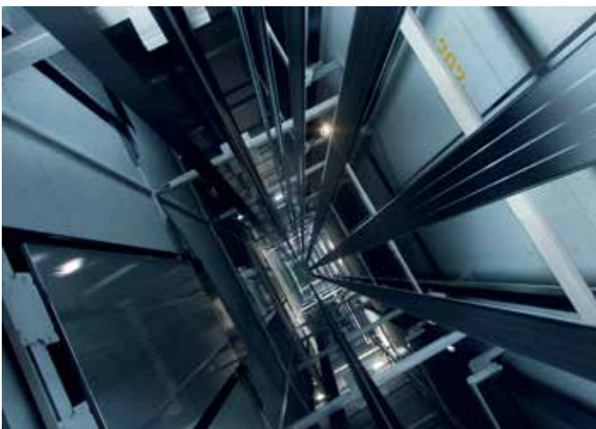
Figure 1. UltraRope, a carbon-fiber and epoxy-based product, is a fraction of the weight of a traditional steel-cored hoisting rope. © KONE
