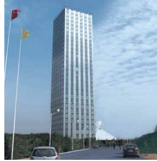
Figure 4. The T30 tower, Changsha, was constructed in 15 days using a custom prefabrication system. © Broad Group
