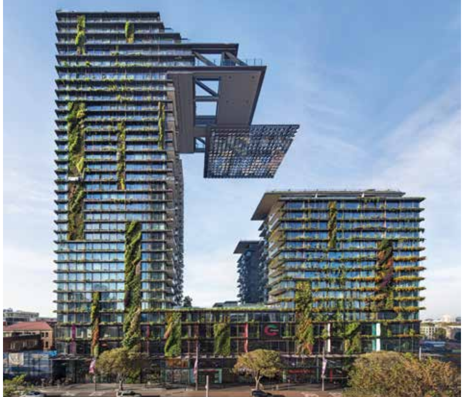
Figure 15. One Central Park, Sydney, used "Living Walls" – vegetation – as a critical part of its façade strategy. © Rob Deutscher
