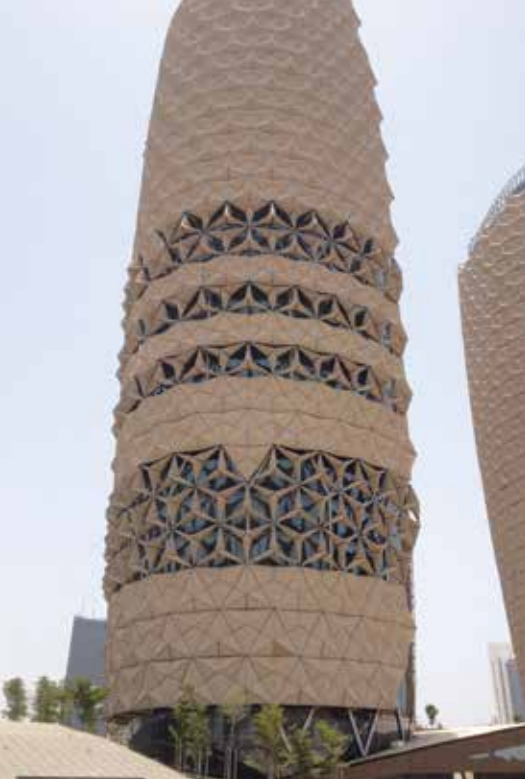
Figure 12. The operable façade of Al Bahar Towers protects the building from harsh sun and blowing sand, while lending it a regionally specific identity. © Aedas
