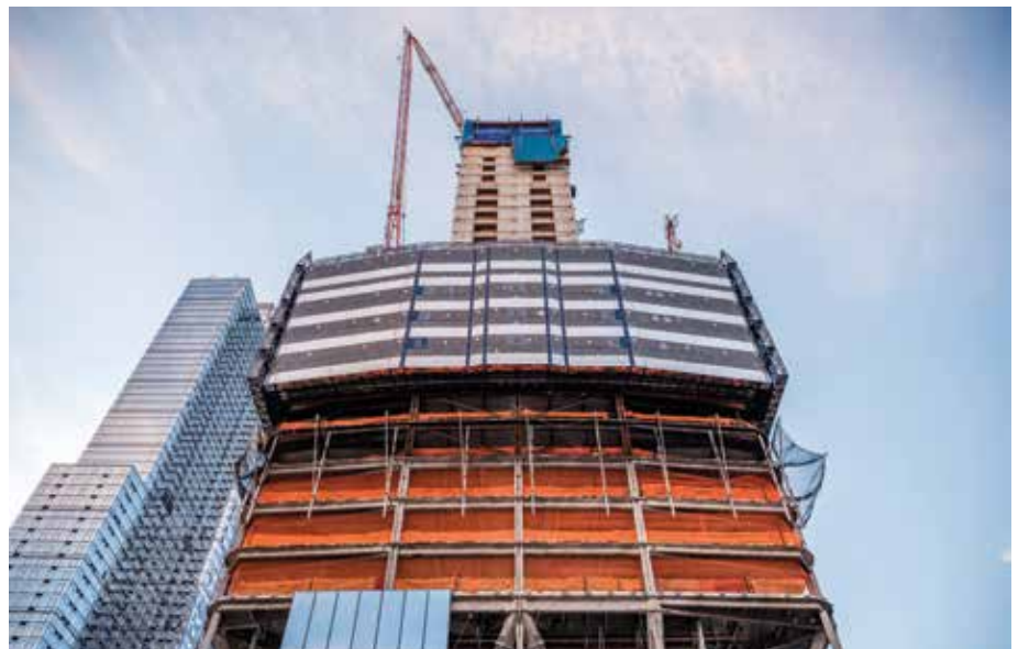
Figure 10. The Self-Climbing Kokoon advances up the core of One Manhattan West, New York. © Despe S.p.A
