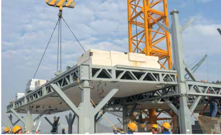
Figure 3. The BSB prefabricated system is assembled at the company's test site in Changsha. © Broad Group
