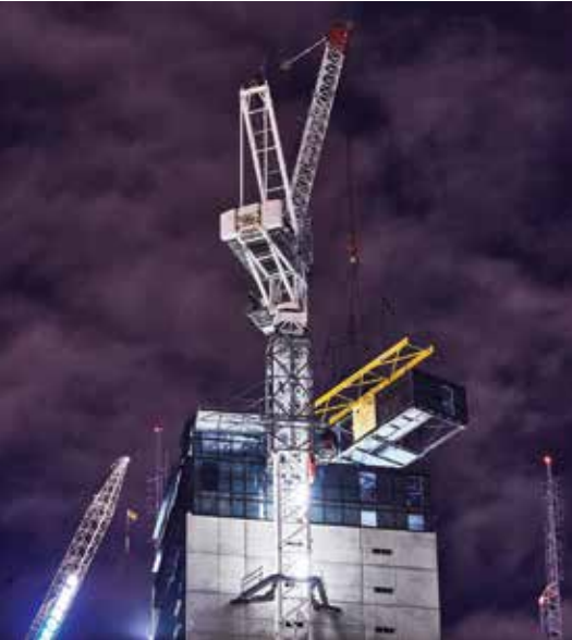
Figure 5. The Atira La Trobe apartments in Melbourne used prefabrication and nighttime construction to minimize disruption to its city-center neighbors. © Hickory Group
