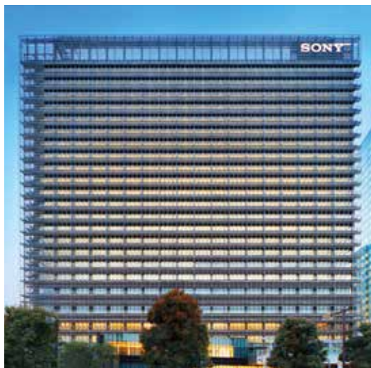
Figure 13. An elevation view of the NBF Osaki Building, with its ceramic perimeter façade. © Harunori Noda
