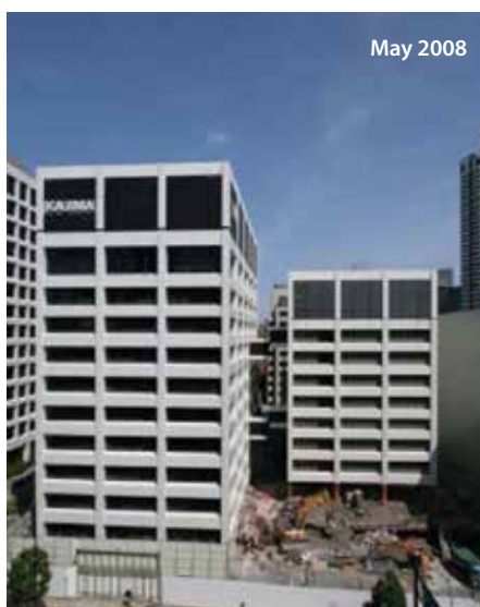
Figure 11. Kajima Cut & Take Down (C&TD) method, used on Kajima's former headquarters in Tokyo. © Kajima
