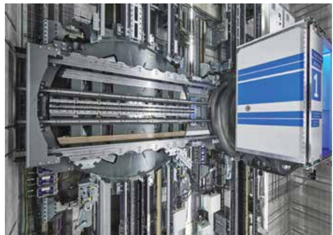
Figure 2. In the MULTI ropeless elevator system, “exchangers” transfer cars from one shaft to the other, or divert their path of travel. © thyssenkrupp
