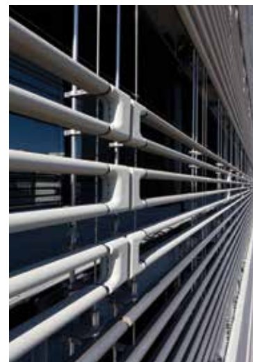
Figure 14. A close-up view of the ceramic transpiration system built into the NBF Osaki façade, known as BioSkin. © Harunori Noda
