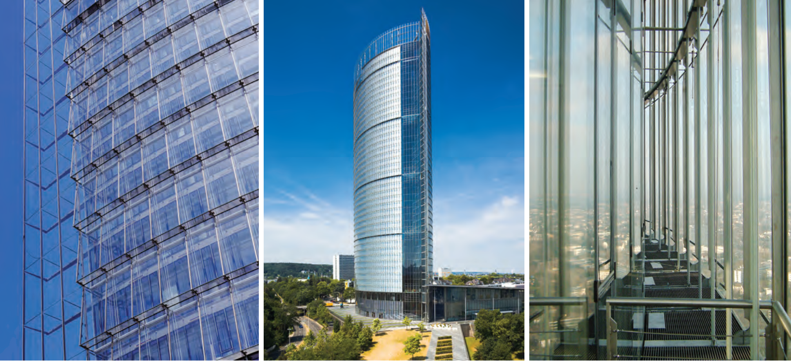
Figure 1. Permeable façade of the Post Tower, Bonn. © Left & Right: Murphy/Jahn; Center: Rainer Viertlboeck
