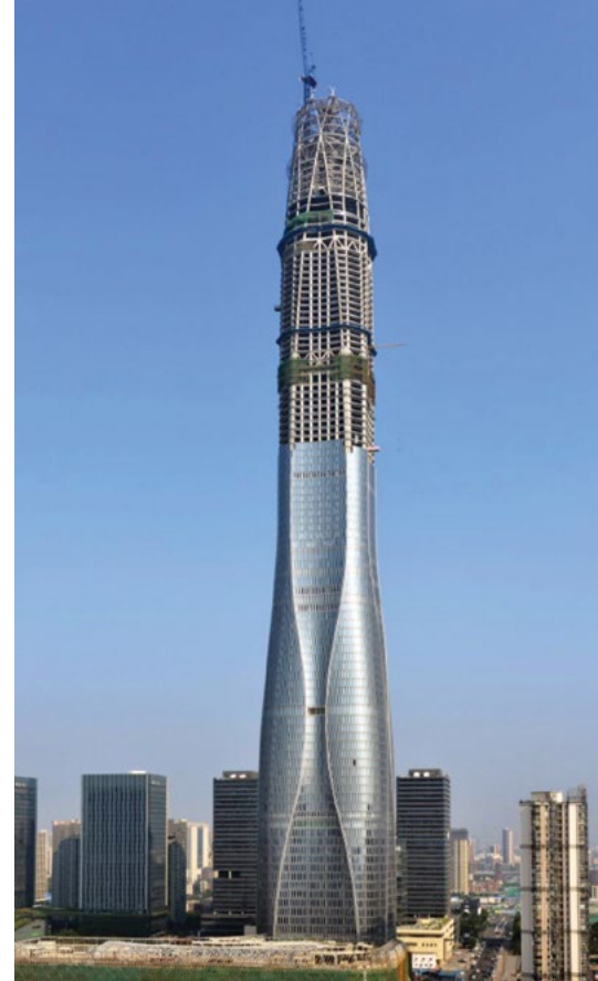
Figure 9. A view of the Tianjin CTF Finance Centre under construction, revealing the integration of envelope and structure. © New World Development
