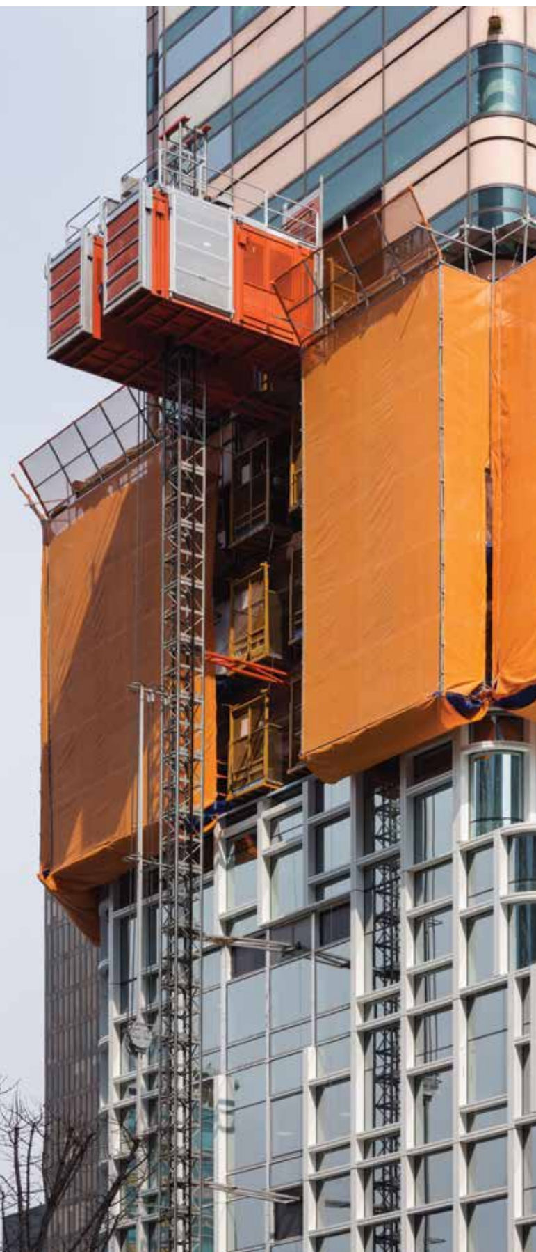
Figure 8. Construction method of refurbishing the building upwards with ongoing works at three floors at a time. © Rohspace
