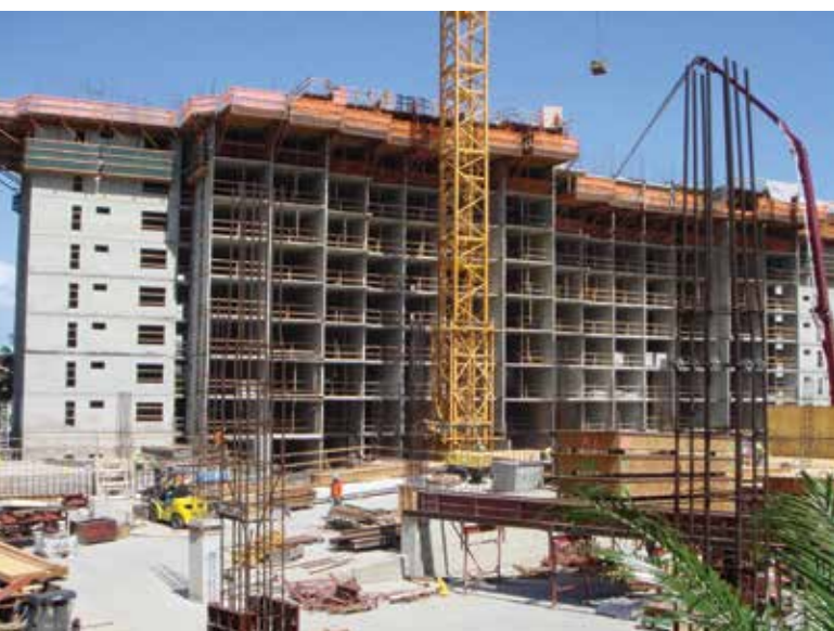
Figure 5. Affordable tunnel form tower under construction uses poured concrete walls, which are erected quickly and create a durable unit. © Steven Baldrige
