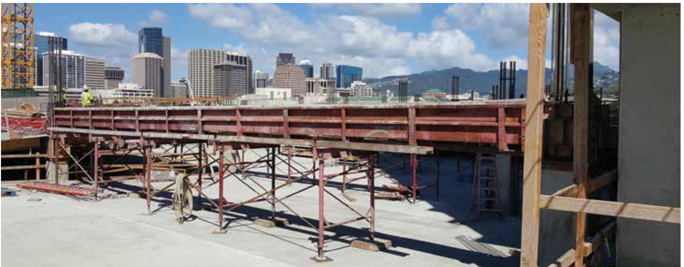
Figure 6. Garage beam steel forms can be moved easily, cutting down on costly crane operations. © Steven Baldridge
