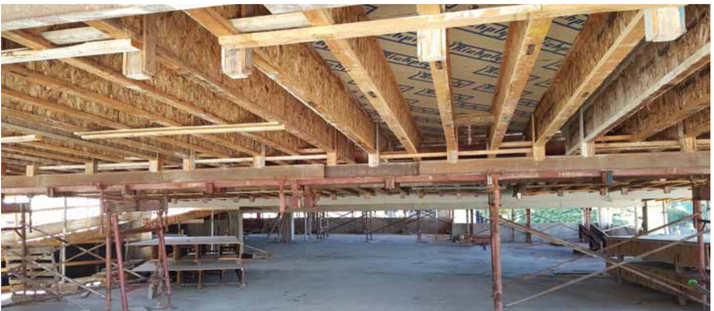
Figure 7. Garage slab form panels can also be moved relatively easily up parking structure ramps. © Steven Baldridge
