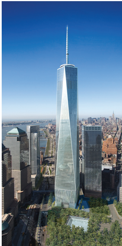
Figure 7. One World Trade Center, New York City, was originally conceived with an enclosure around its topmost projection, making the object more easily identifiable as a “spire” (left). CTBUH eventually ruled that the object as completed (right) was indeed a spire, giving it a 541-meter height and current rank as world’s sixth-tallest building. © Skidmore Owings & Merrill/dBox (left); Pedro Szekely (cc by-sa) (right)
