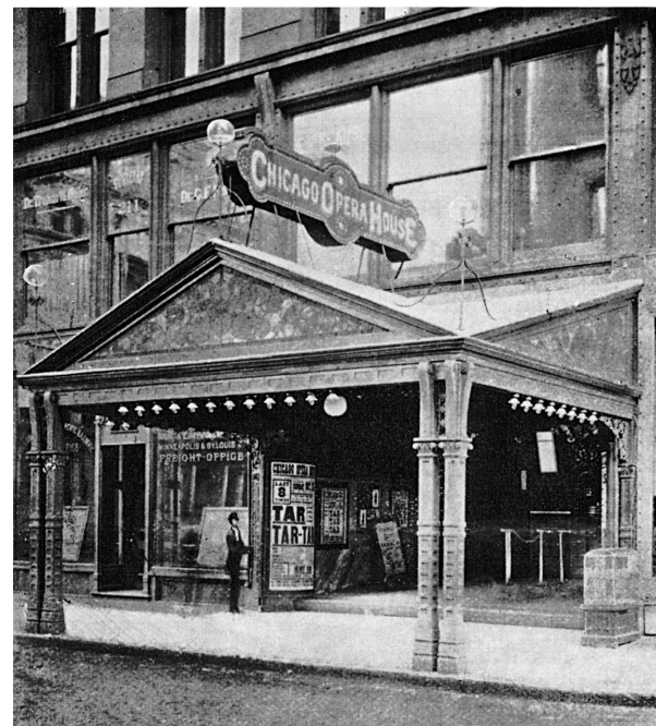
Figure 31. Cobb and Frost, Chicago Opera House Block, Detail of exposed iron framing in the first two floors. (Siry, Auditorium .)
