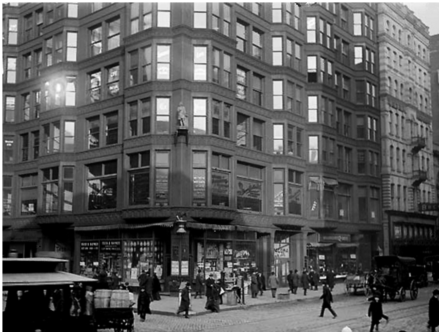
Figure 49. Holabird and Roche, Tacoma Building. Note the large plate glass windows in the second floor. ( http://connectingthewindycity.com )
