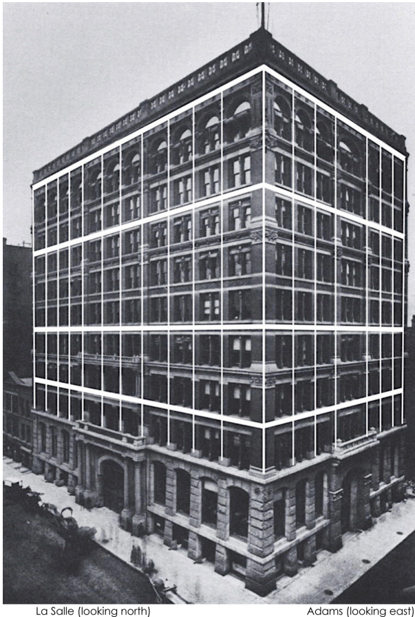
Figure 39. Jenney, Home Insurance Building. The exterior iron structure overlaid the building's elevations, showing the lack of spandrel beams in Floors 5, 7, 8, and 10. (Drawing by David Burwink.)
