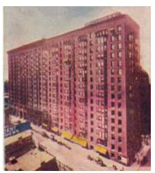
Figure 3. View from northeast showing masonry bearing walls and cantilevered bay windows. Source: Contemporary post card, author's collection
